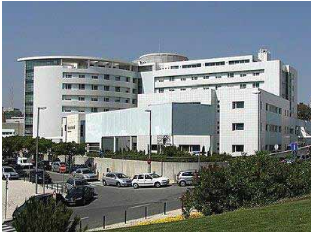
Facilities of CUF Descobertas Hospital
